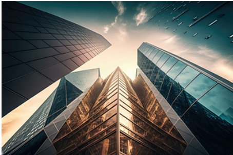
Pressure boosting in tall buildings
