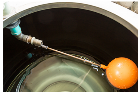
Level control float switch
